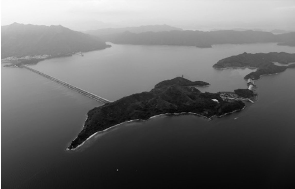
Figure 5.4. Aerial view of Plover Cove Reservoir. (Photograph by Dorothy Tang.)
