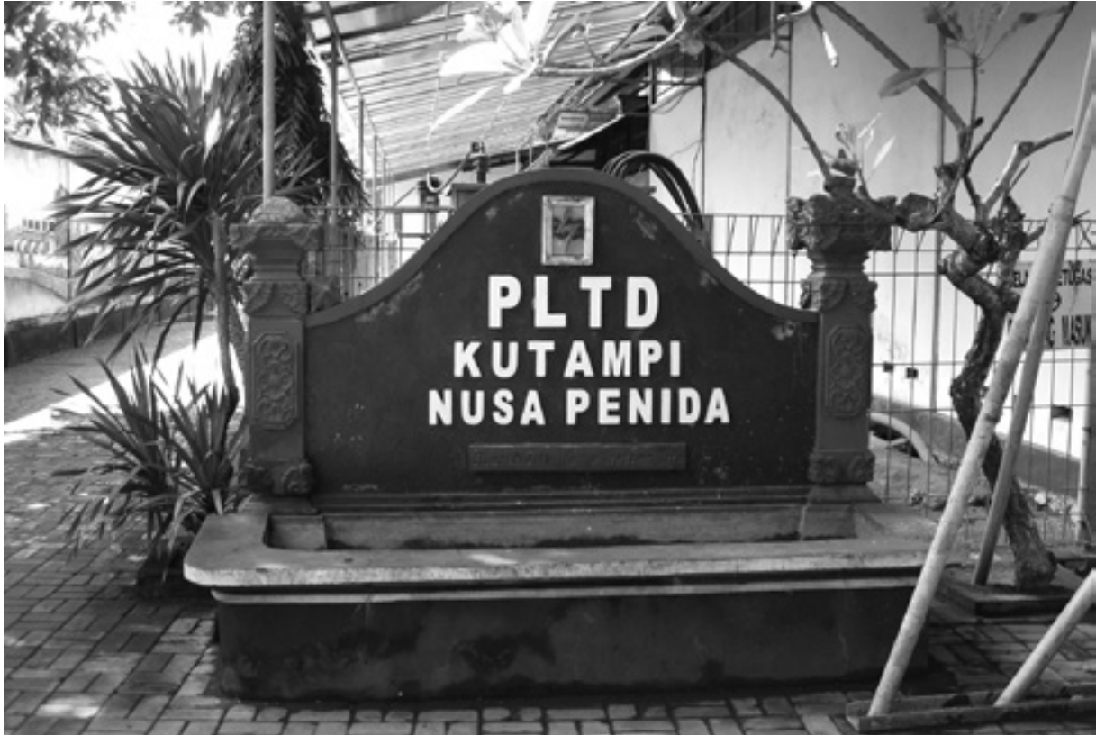
Figure 4.2. Kutampi Diesel Power Station, in Nusa Penida. (Photograph by Anto Mohsin.)
